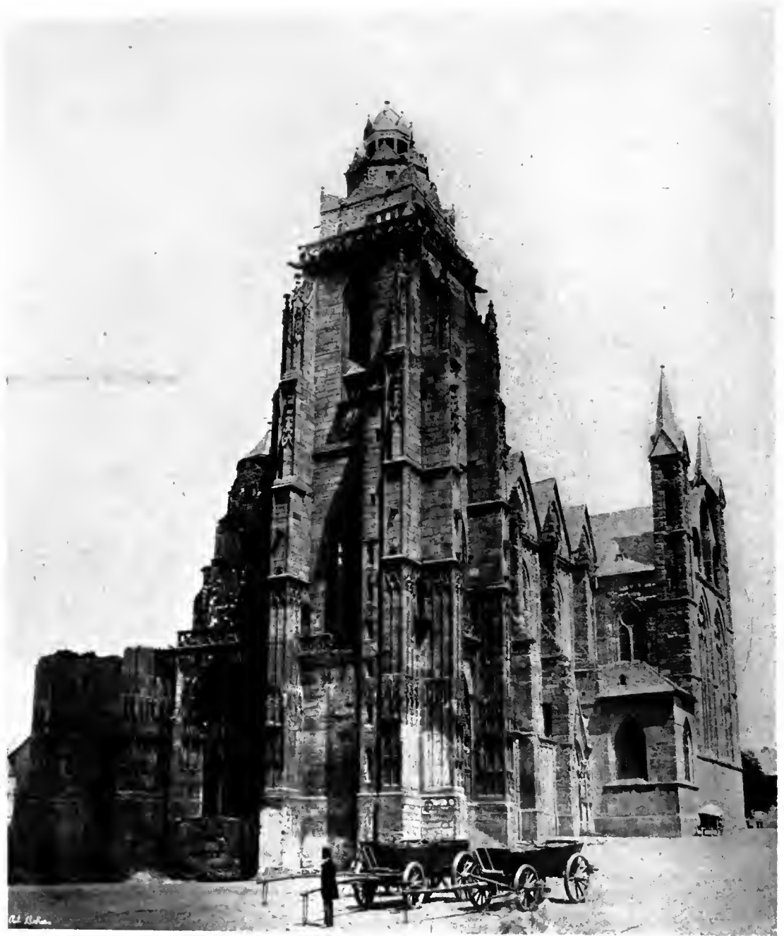
THE CATHEDRAL, WETZLAR, GERMANY
